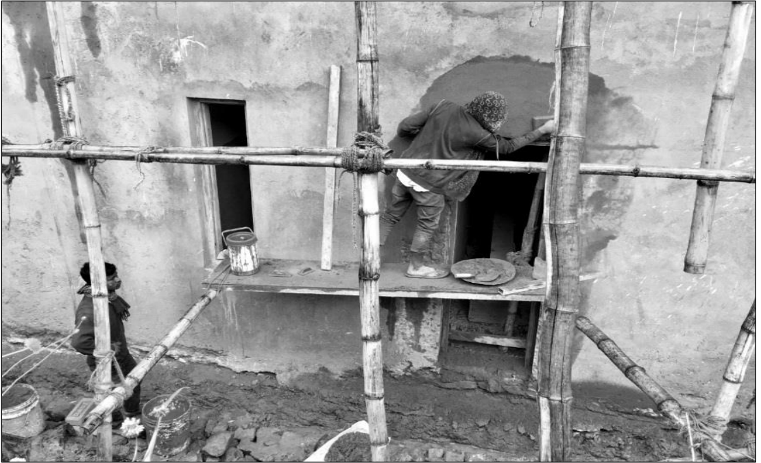
Fig. 2: A construction worker at work. (Photo: Author)
