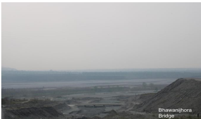
Figure 5: Bhawanijhora Bridge and environmental precarity in Pasakha. Photo
